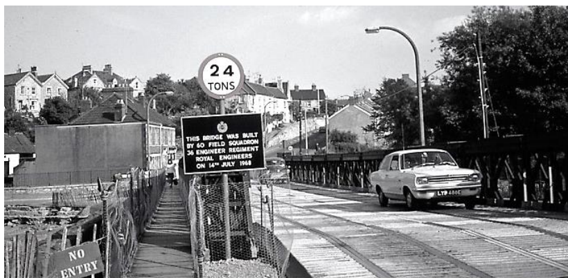
The temporary Bailey bridge at Bath Hill built by the Royal Engineers on 14th July 1968 (Photo from the Russell Leitch collection)
